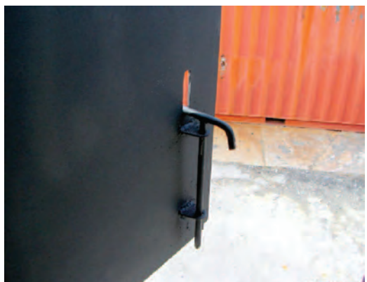
Figure C-6: Window & Latch Construction
