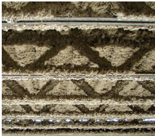
Figure C-4: Fireproofing added to structural steel
