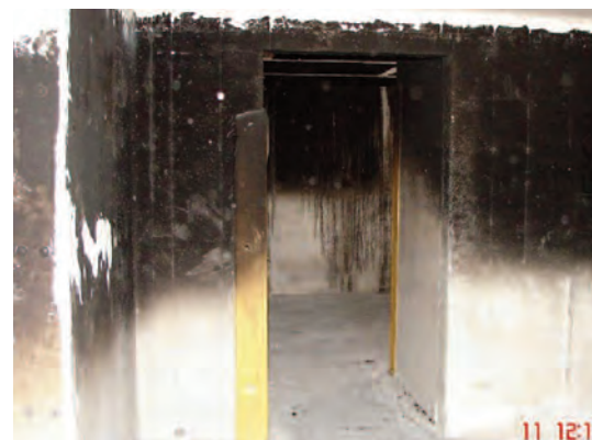
Figure C-7: Interior View of Burn Prop
